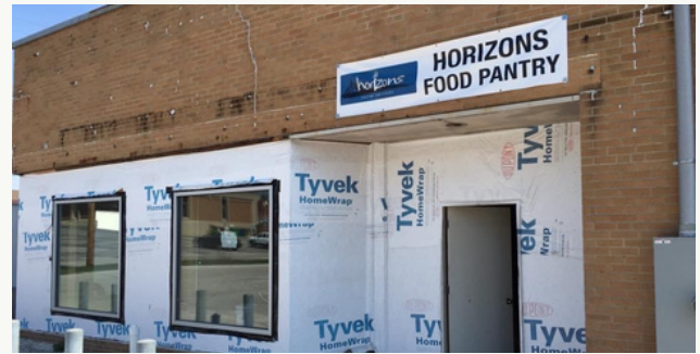
Renovations of the new Horizons location
